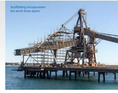
The second shutdown started in late-October. Local company South East Scaffolding erected 110 tonnes of scaffolding to encapsulate the ship loader boom and capture sandblasted debris. It took five days to erect and five days to pull down when the work was completed; a great example of the Port and a professional local company working together to achieve a positive outcome.
