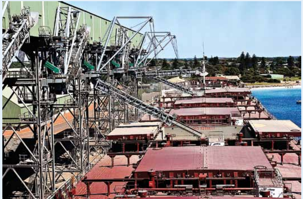
Above: Deck view of loading operations on Berth 1.
