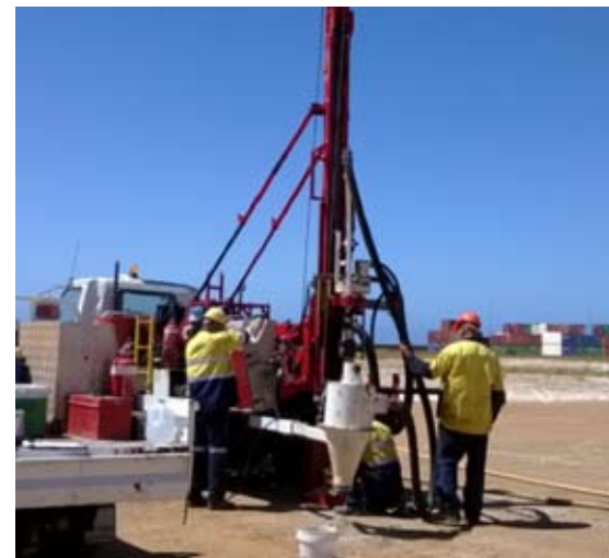
Coring activities on the reclaim area
