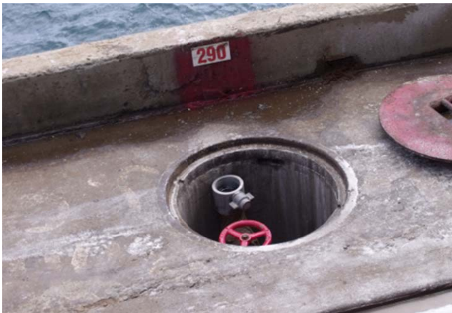
Figure 8. Water hydrant 290 used for washdown
