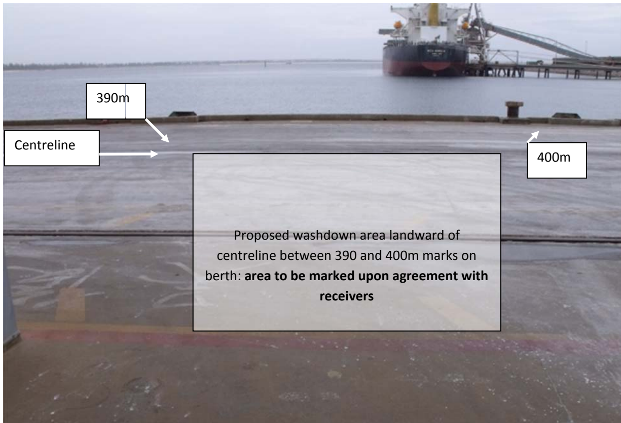
Figure 6. Alignment of hopper washdown between 390 to 400m mark on berth 2, landward of berth centreline. The area seaward of centreline should be kept clear to allow Environmental Services to sweep up any spills from the containment used to capture hopper washings. Ensure all services lids are sealed in this area.
